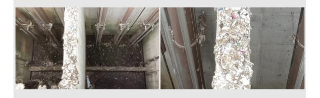
Chuck explained that this slide shows where all the wastewater from the city comes into the Wastewater Plant. The debris shown in the picture is mostly the wipes that say they
