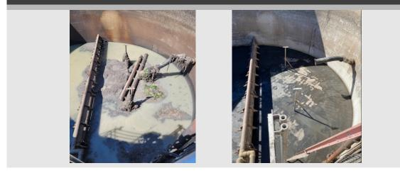
Chuck explained that the picture on the left is SBR#3 before it was cleaned out and the one on the right is after it was cleaned out and before the decanter was put back in.
