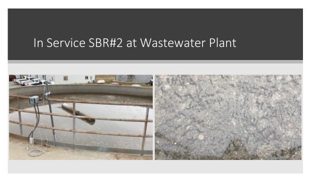
This slide shows SBR#2 that is currently running in good condition but has a lot of debris on the surface that will make it through the current bar screen.
